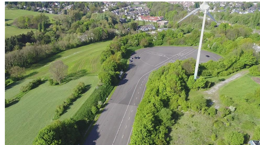
Acoustic road surface (DIN ISO 10844/94) width 20 m; length 45 m
